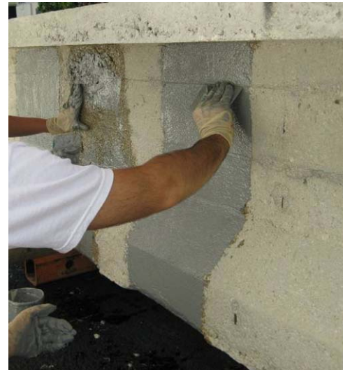
Figure 5.1 – Application of Primer Figure 5.2 – Application of Putty
