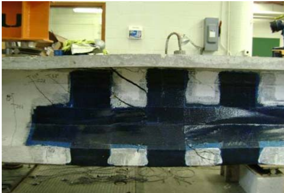
Figure 7.25 – B-3a Failed Section 1
