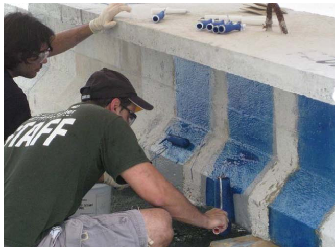
Figure 5.3 – Application of Saturant
